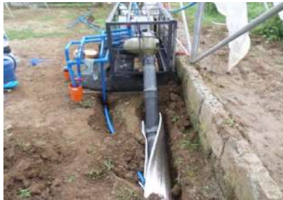
A - Water pump and Blower
