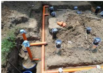
E - return pipes of the nutrient solution
