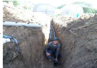
B - buried pipes for air and water flow
