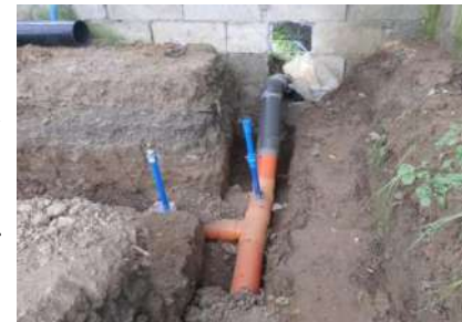
C - distribution line for air flow to the aeroponic tower
