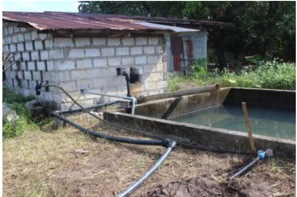
Separate mainlines for drip and furrow irrigation system
