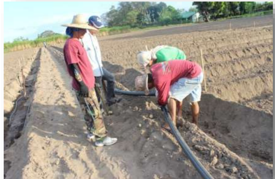
Installation of 63 mm HDPE mainline for furrow irrigation
